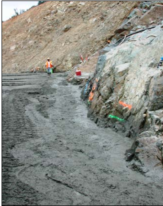
Completed Grout Enriched RCC at abutment
